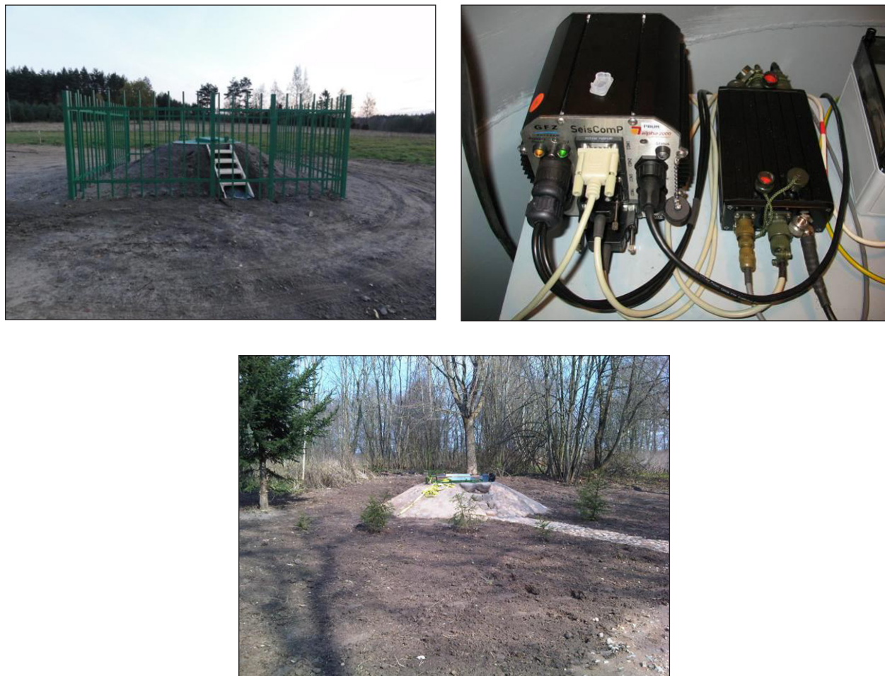
Fig. 3. Vaults of: (a) Paburgė and (c) Paberžė seismic stations (author A. Pačėsa); (b) seismometers installed in both seismic stations (author J. Čyžienė)
