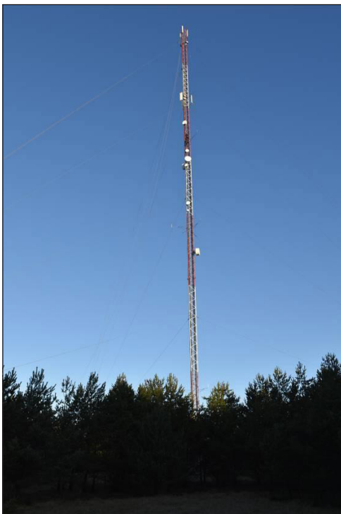
Fig. 5. Guyed type lattice triangular mast, which has a height of about 100 m with the side width of 1.2 m
