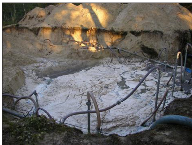
Fig. 2. High level of shallow groundwater at excavated site near the boreholes field
